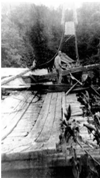
The old suspension bridge collapsed in about 1954.
