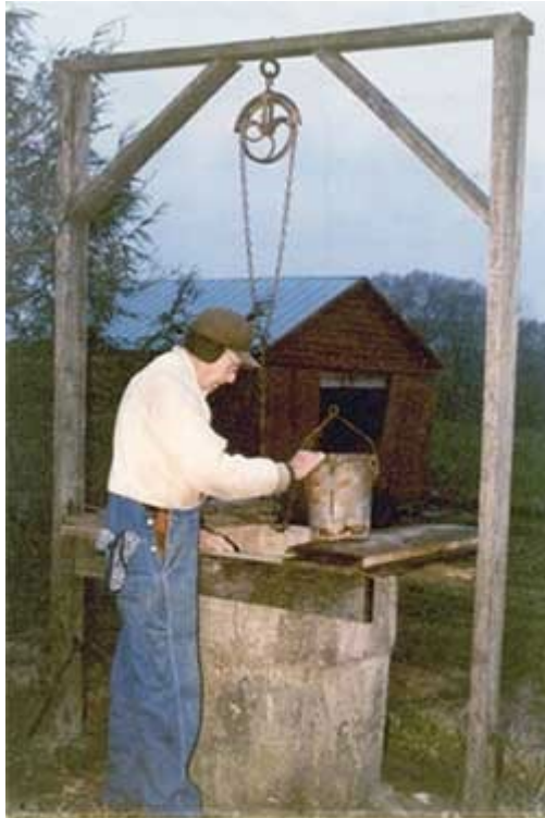
This is not our well, but serves to illustrate the general idea. Our pulley looked like this, but we had no circular concrete surrounding the hole in the ground. The hole into which we lowered the bucket (see the photo to the right), was about 8 to 10 inches in diameter.
