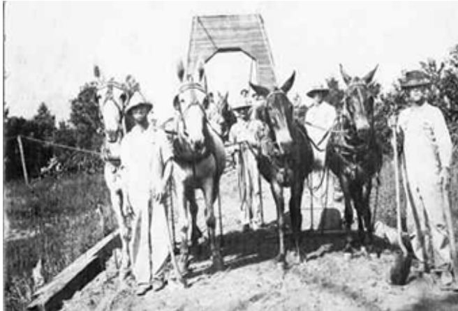
The bridge, under construction, in 1909. formed the roadway for the wheels of the wagon or car.
